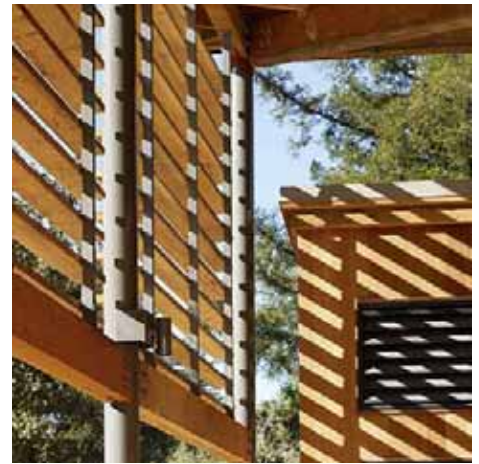
Solar control devices should not interfere with the transparency of a building facade.
