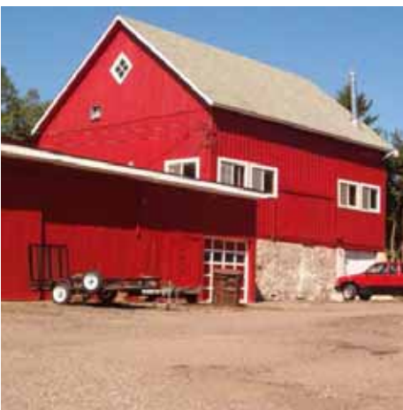
Exterior building material should convey a sense of integrity, permanence and durability.
