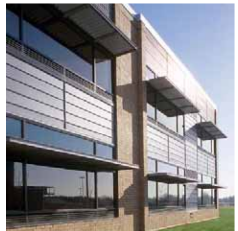
Protect all glass areas exposed in summer with deep recesses, overhangs, or other devices to minimize heat gain.
