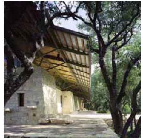
Solar control devices should not obstruct views into and out of the building.
